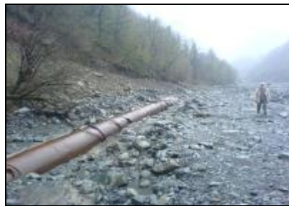
Penstock (in riverbed)
